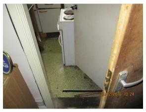
Another example of a fire safety hazard is poor means of escape. The photo below shows the escape route from a flat above a café exiting in the commercial dining area.
